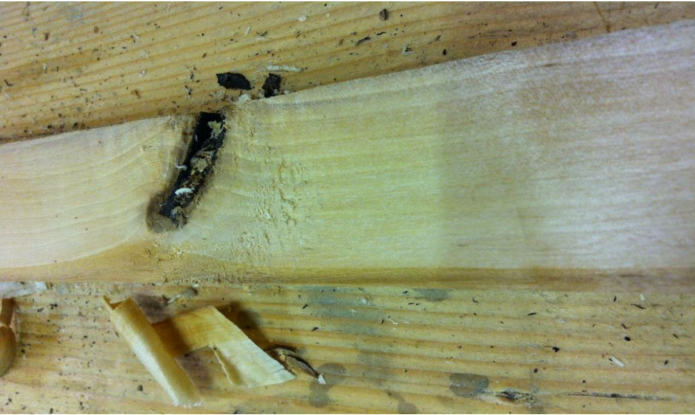
Figure 2 Tearout visible on the right side of the knot.
